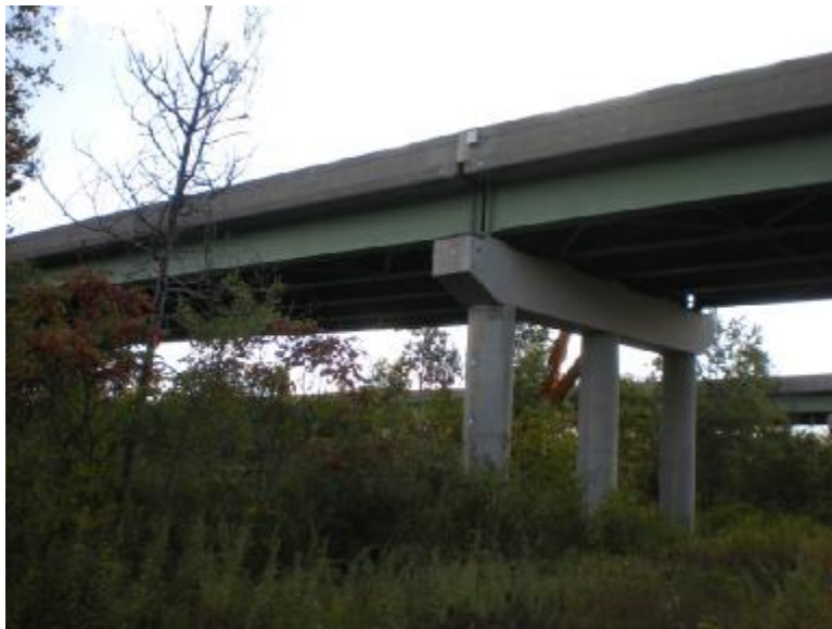
Figure 22. Photograph of pier 3 of the bridge.
