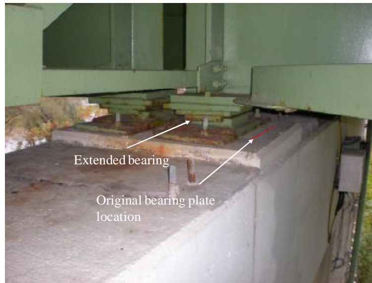
Figure 23. Photograph of expansion device at pier 3.
