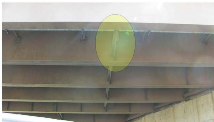
FIGURE 8 Retrofit girder replacement cross frame stiffener measurement locations.
