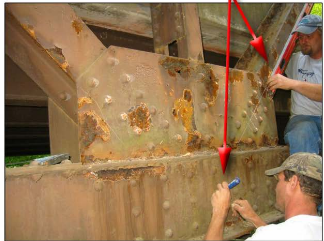
FIGURE 2 Current manual measurements for bridge retrofit work made by hand directly on the structure.
