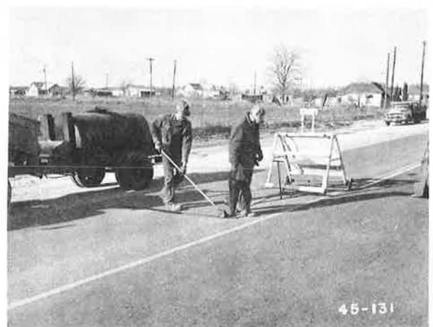
Figure 14. Crack sealing operations in progress.
