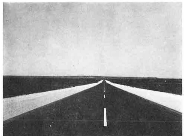
Figure 12. A section of completed highway.
