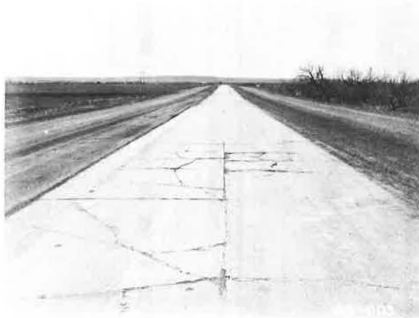
Figure 4. Original pavement condition before it was broken up and recompactd.
