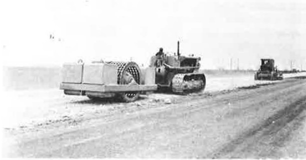
Figure 9. Grid roller used in the compaction process.
