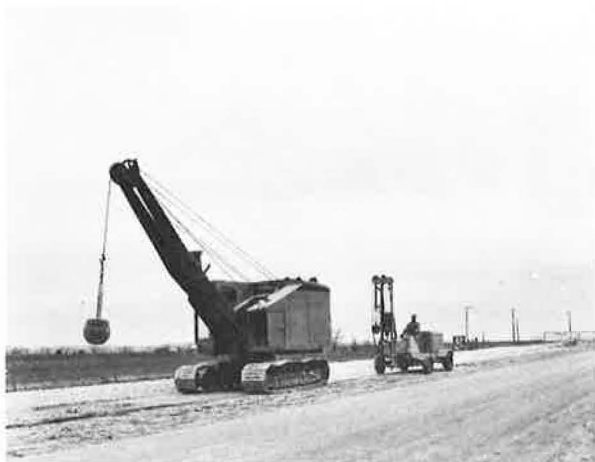
Figure 6. Machinery used in breaking up and compacting old concrete.
