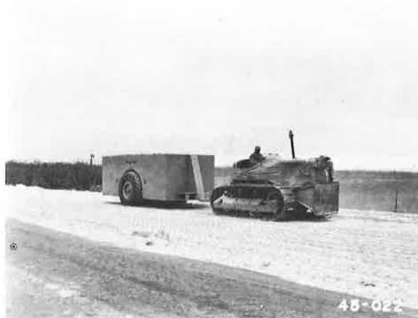
Figure 7. Machinery used in breaking up and compacting old concrete.
