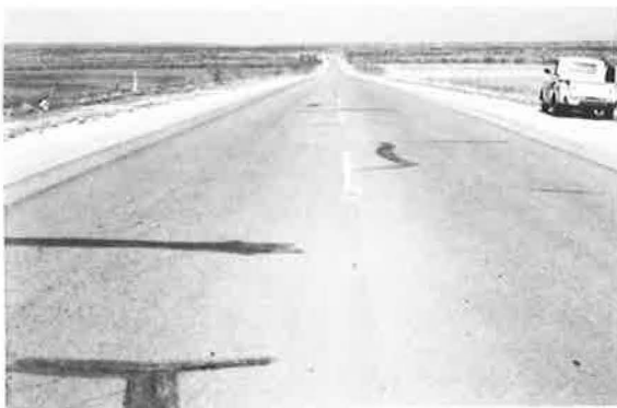
Figure 21. The general condition of design section No. 3 in 1961.
