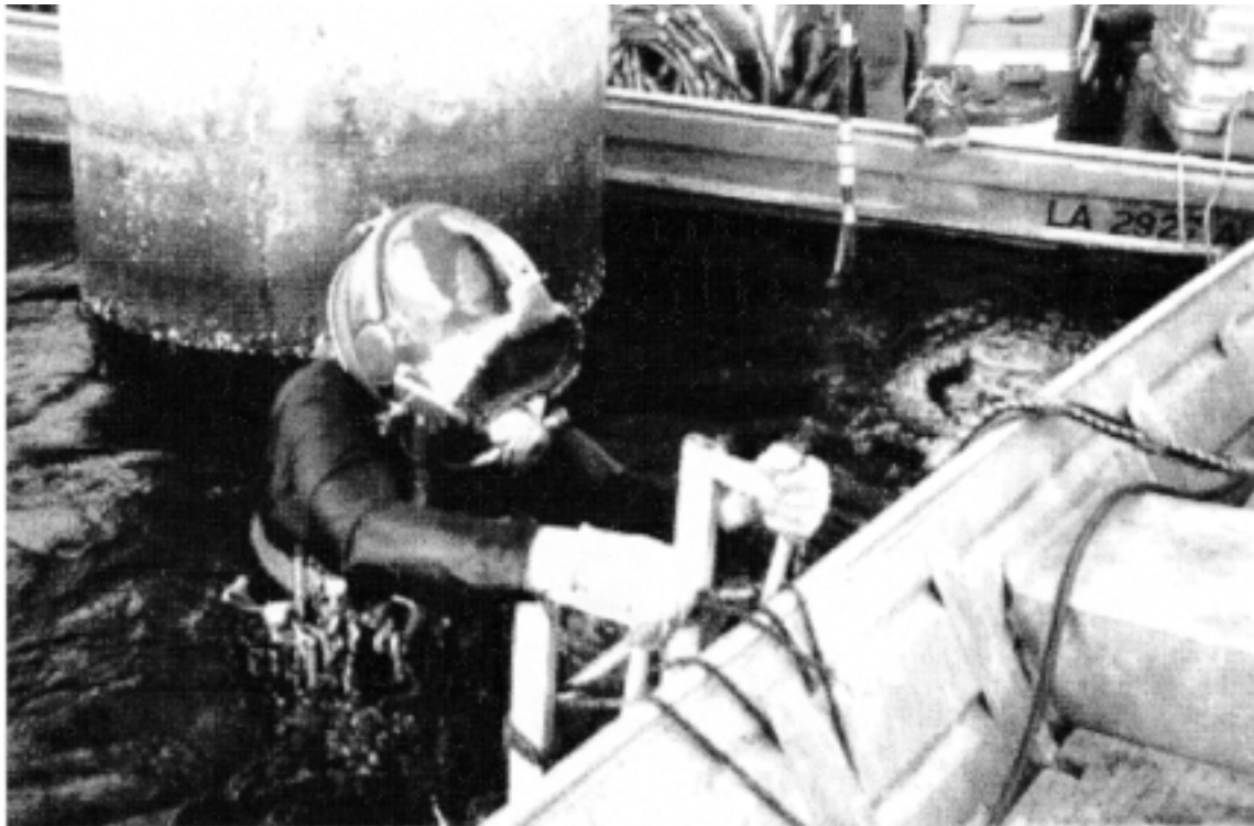
Figure 1: Underwater dive inspector.
