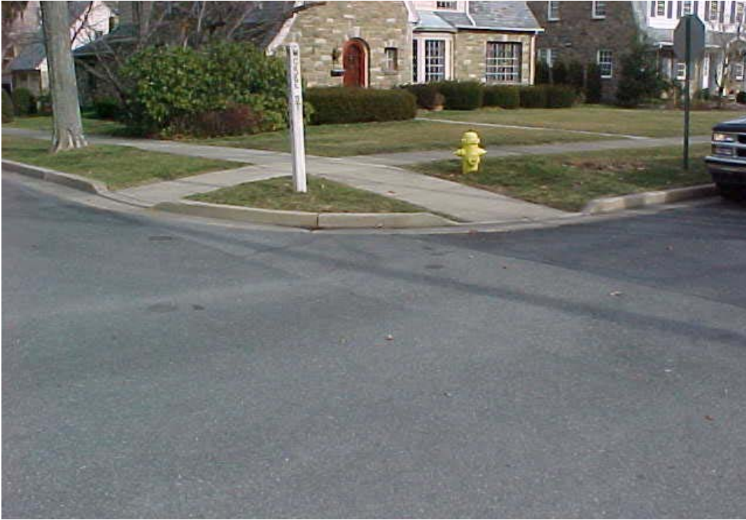
FIGURE 3 Residential street in State College exhibiting treated versus non-treated pavement.
