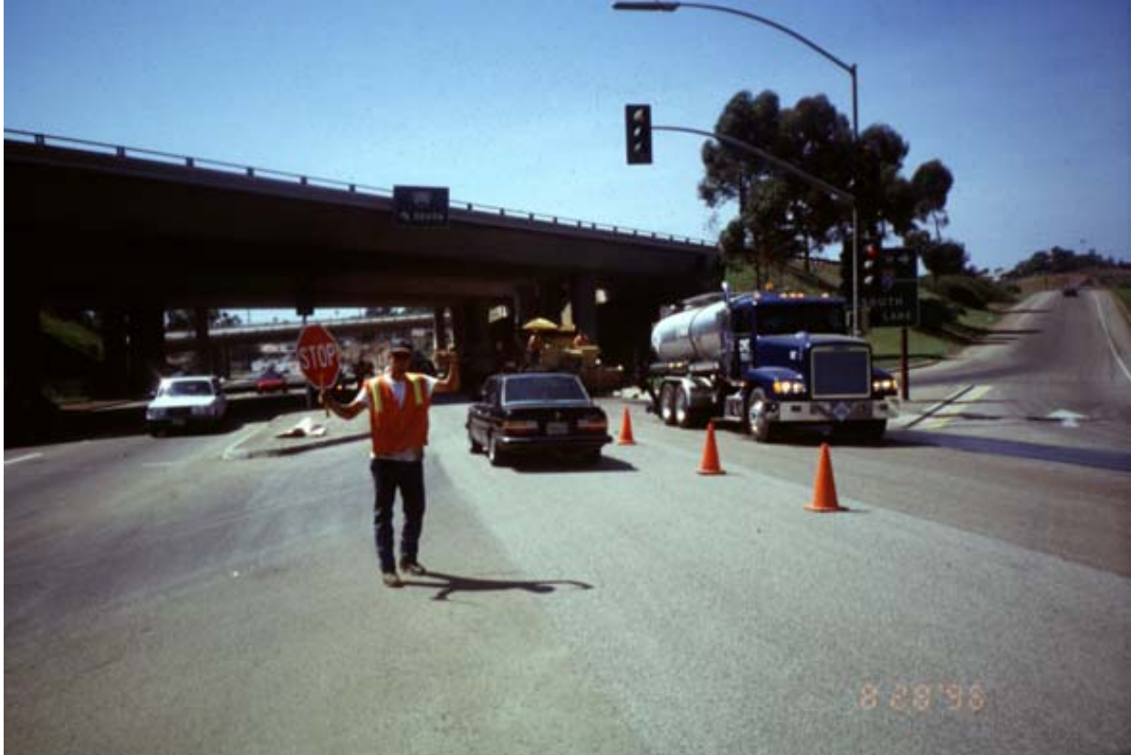
FIGURE 2 Maintain low traffic speeds to prevent damage to the chip seal and windshields.
