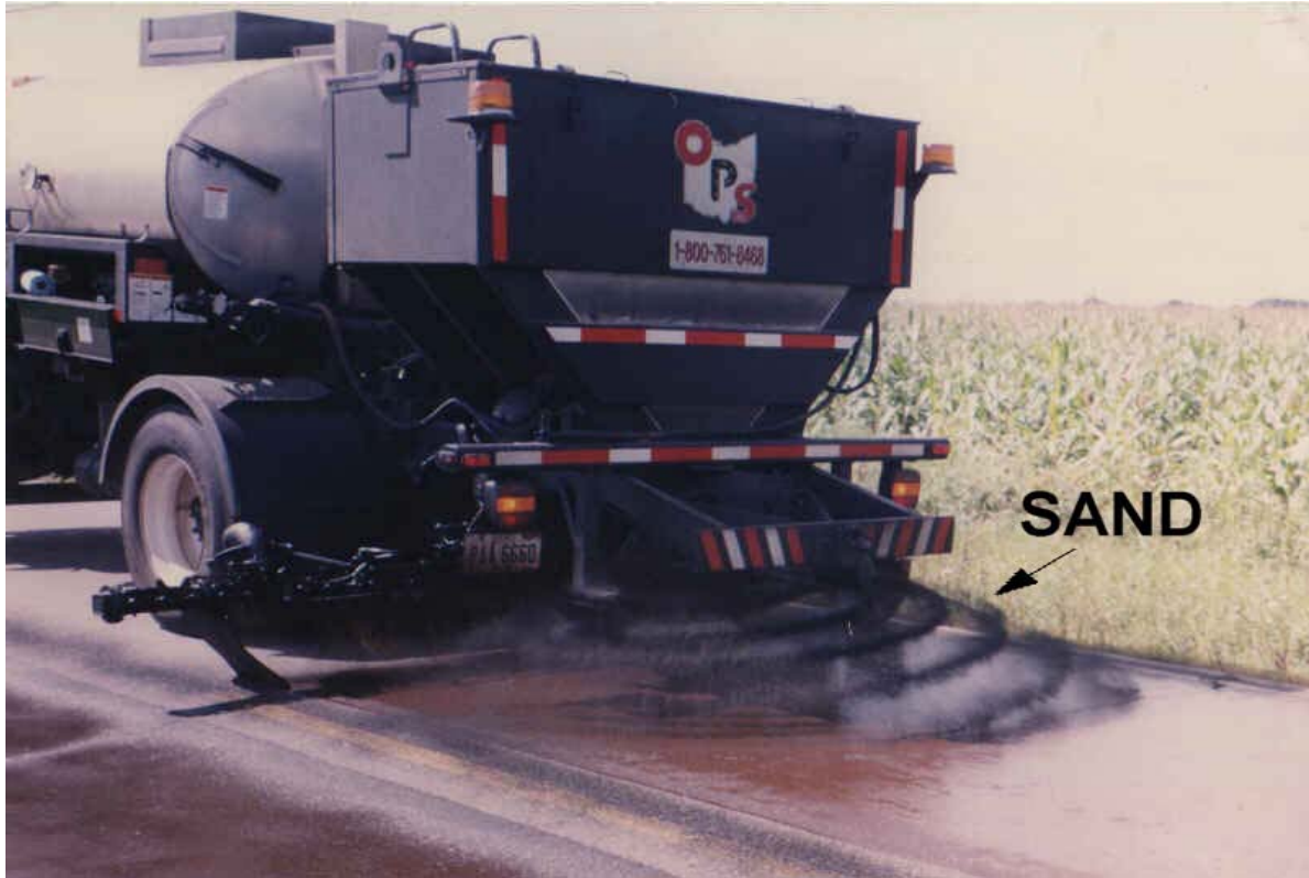
FIGURE 2 Asphalt emulsion distributor equipped with sand hopper for one-pass application.
