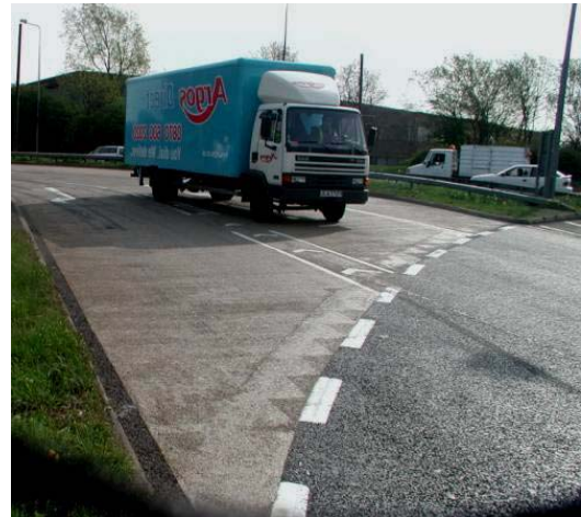
Figure 16 - Shell-coat Skid Treatment
