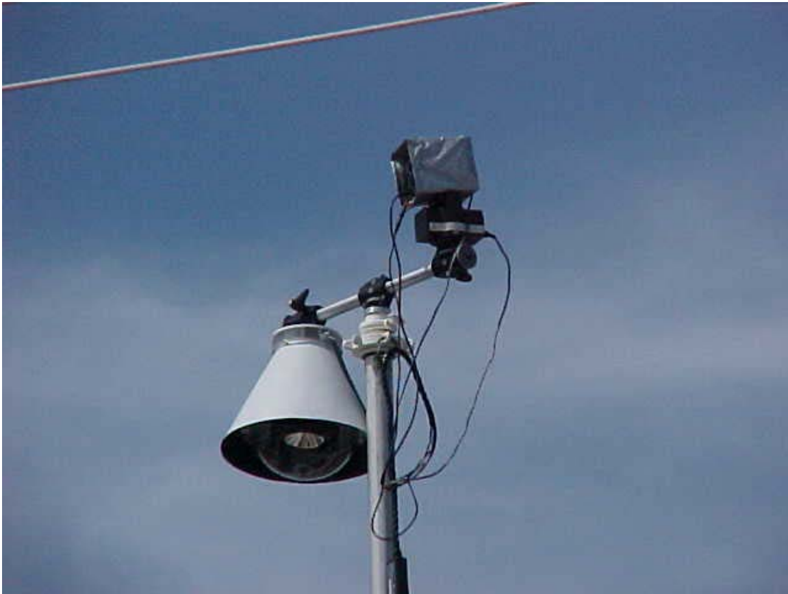
Figure 3. Omni-directional camera and digital camera located at top of mast
