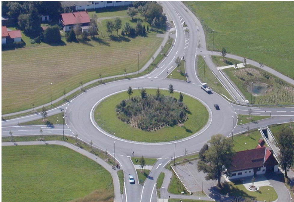
Fig. 8: Rural compact two-lane roundabout in Bad Aibling
