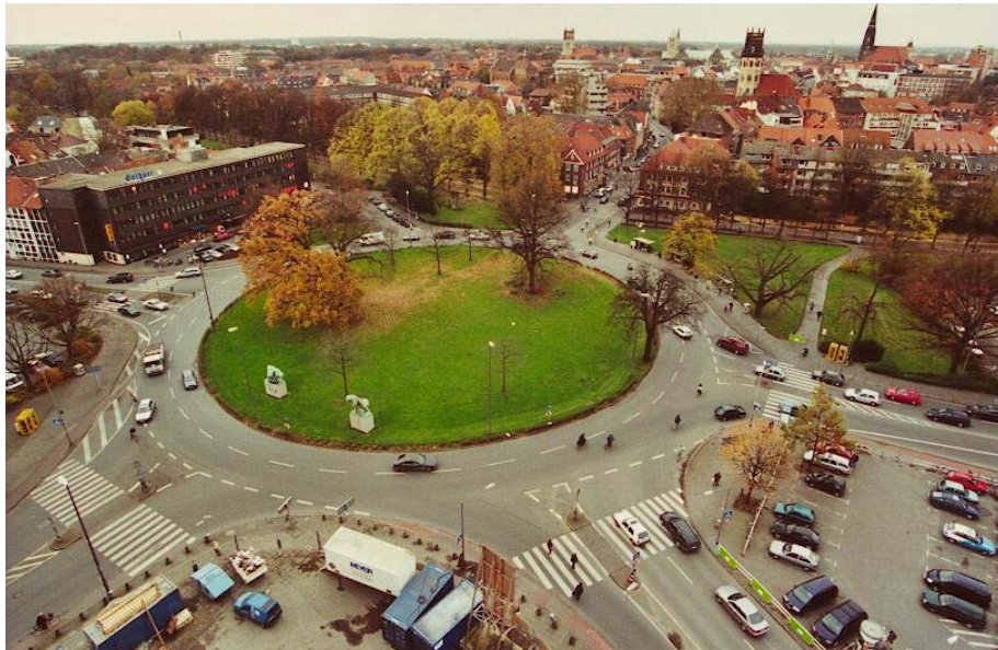
Fig. 1 : Large traditional roundabout: Ludgeriplatz in Muenster
