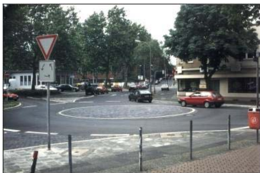
Fig. 4: Mini roundabout in Bochum built by a reconstruction of the intersection
