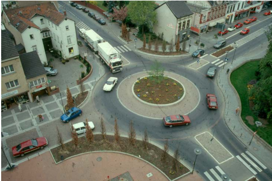
Fig. 5: Compact single-lane roundabout in the town of Bruehl (near Cologne) with a paved apron at the inner side of the circle (Photo: Nikolaus, Euskirchen)
