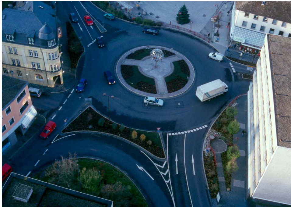
Fig. 7: Urban compact two-lane roundabout in Idar-Oberstein
