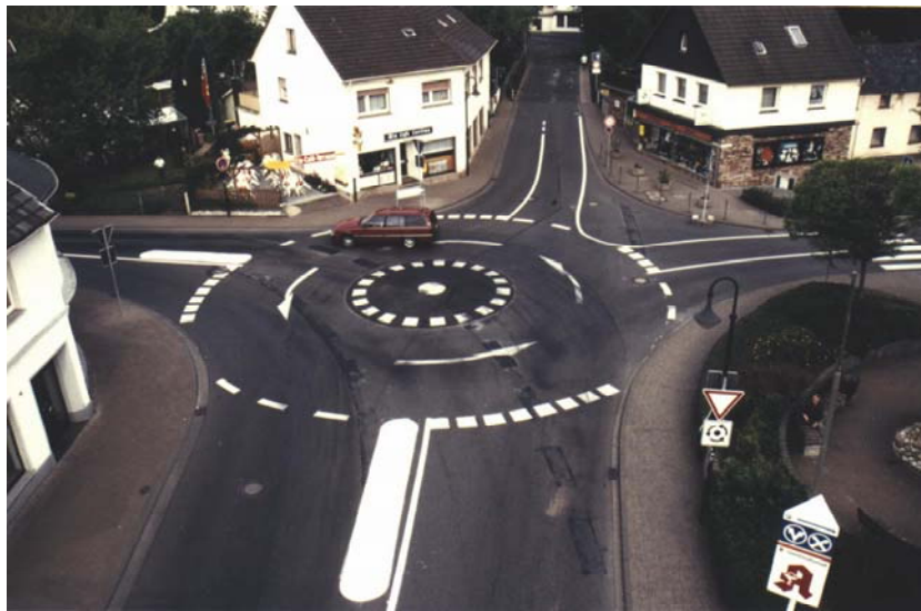
Fig. 3: Mini-Roundabout in Kall built with nearly zero costs (only some asphalt to construct the central island and road markings)
