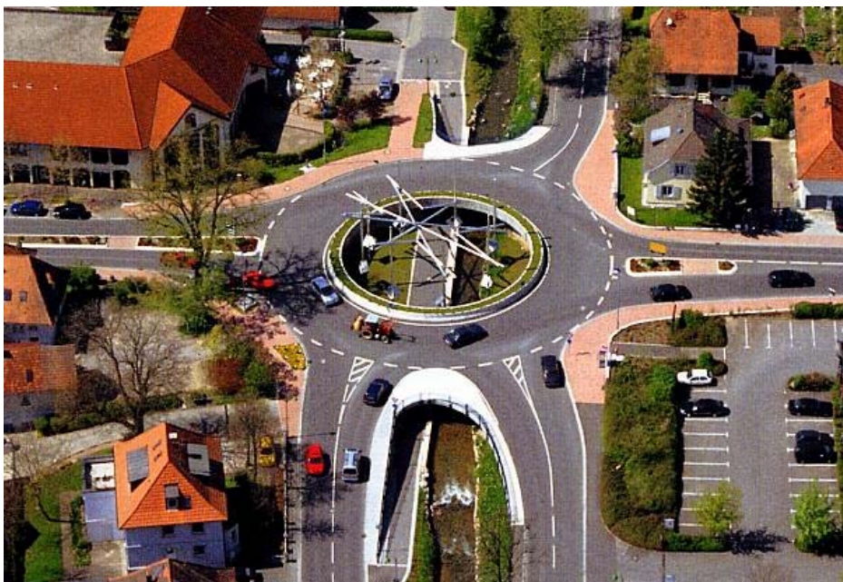
Fig. 6: Urban single lane roundabout built on bridges over a creek (Photo: Lustinez, Freiburg)
