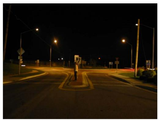
symmetrically around the roundabout as shown in Figure 2. It provides a good illustration of uniform lighting of the circulatory roadway.
