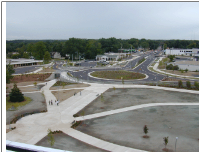
WMU Rbt Pedestrian Underpass to Left
