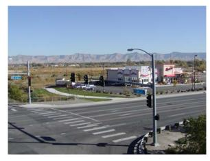
indicated that future traffic volumes would cause congestion. A major drainage channel runs parallel to the east side of 24 Road. Widening the northbound side of the intersection for a right turn lane will require considerable investment to construct a culvert. The projected traffic volumes show that a right turn lane is required in addition to two through lanes.
