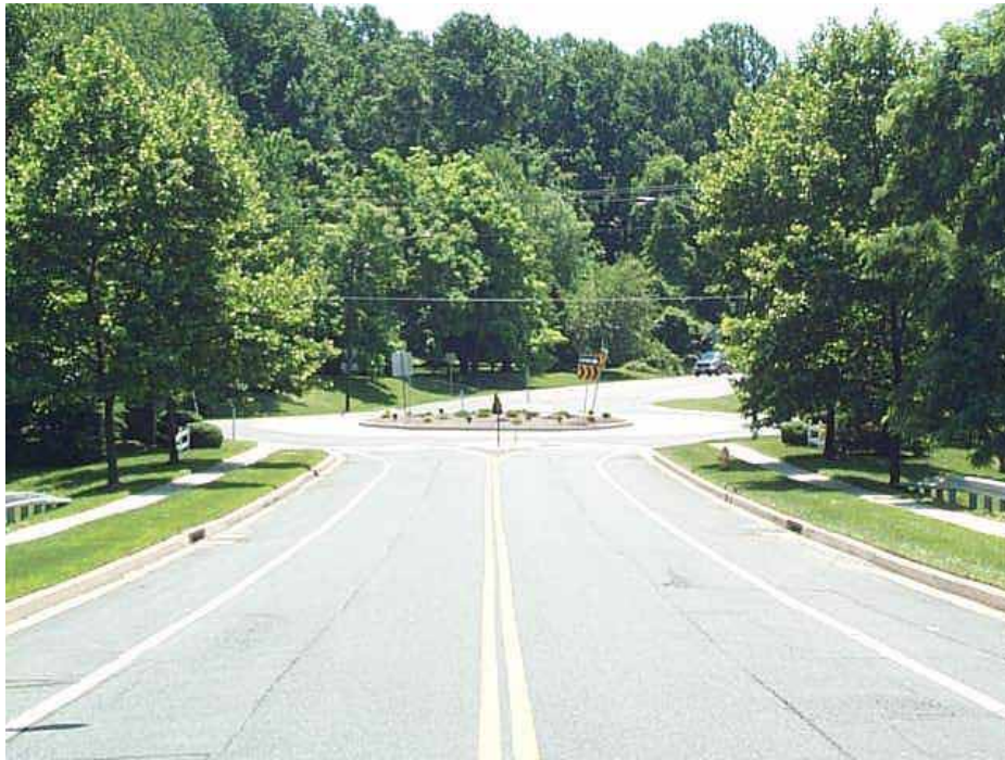
Tollgate Road/Wheel Road Roundabout
