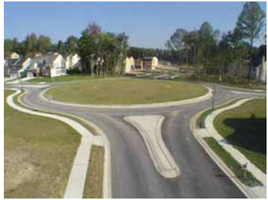
Roundabout currently under construction (Sept. 2004)
