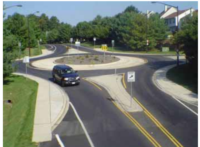
Tollgate Road/Westover Lane Roundabout
