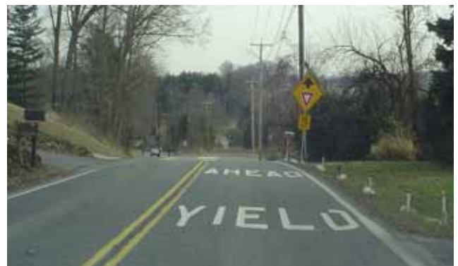
Advanced roadway markings and signing
