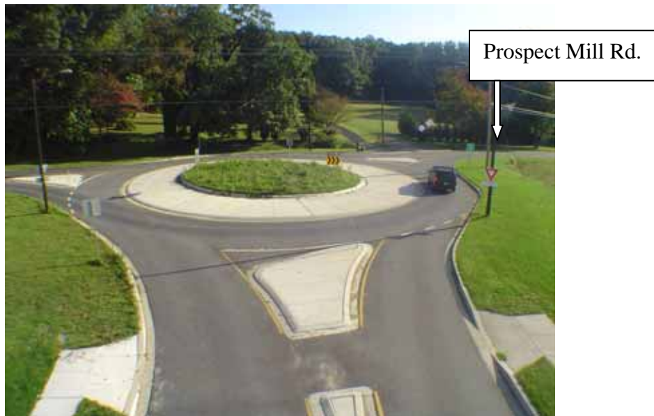
Prospect Mill Road/Wagner Road Roundabout
