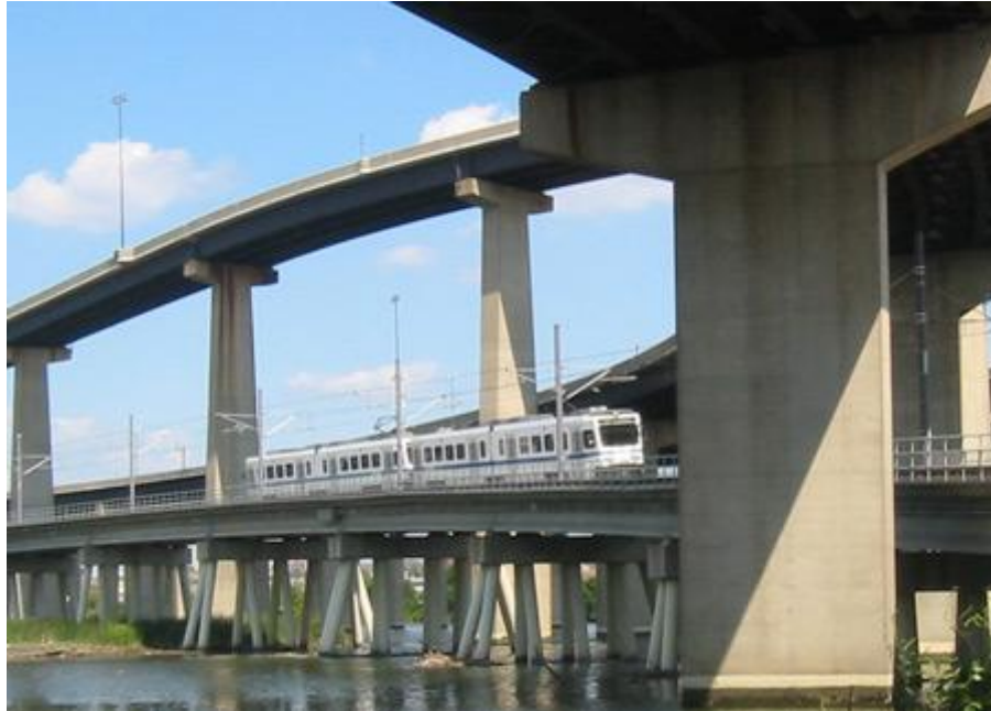
FIGURE 4 MTA CLRL Middle Branch Bridge over the Patapsco River.
