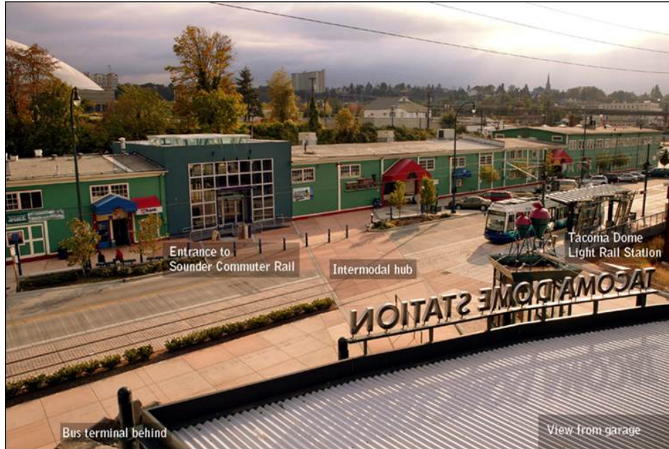
FIGURE 3 Tacoma Link was designed with a stop across a pedestrian-enhanced street from the Sounder commuter rail station. The Tacoma Dome Station park-and-ride garage is also adjacent. The Pierce Transit and Sound Transit bus platform as well as the Greyhound station are directly behind the garage.
