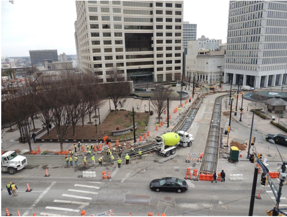
FIGURE 10 In Atlanta construction limits involved substantially less street reconstruction.
