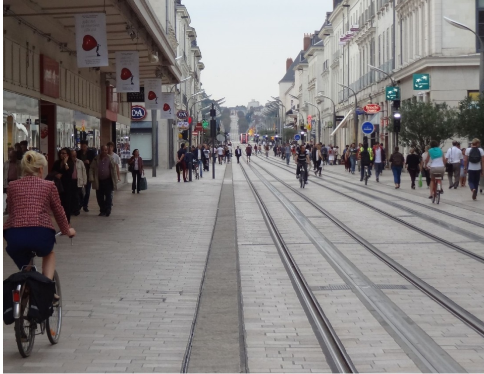
FIGURE 13 Streetcar tracks in a narrow street, National Street, Tours.
