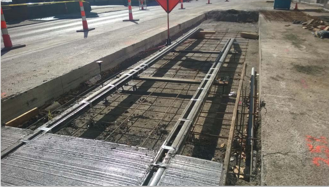
FIGURE 6 112TRAM installation: Kansas City.
