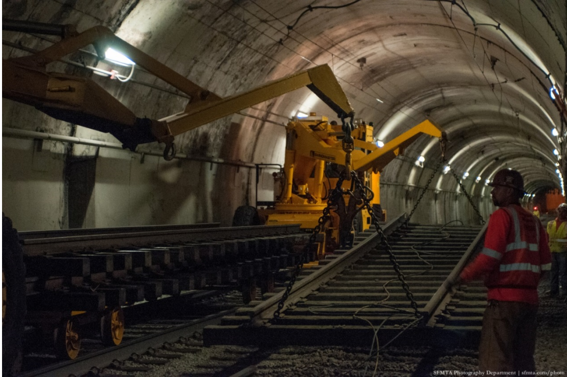
FIGURE 10 Sunset Tunnel construction.
