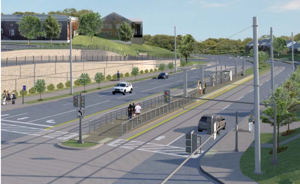
FIGURE 3 Dale Drive Station showing rumble strip at platform.
