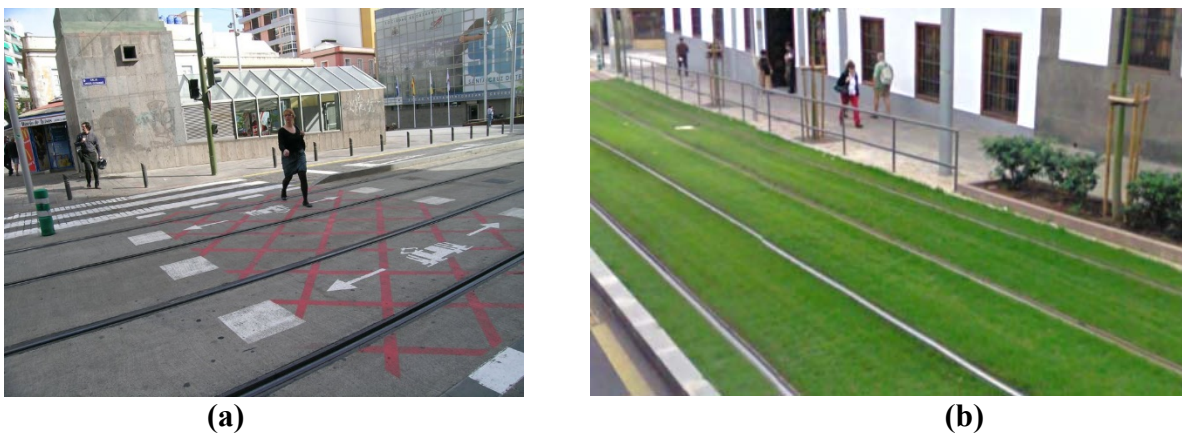
FIGURE 2 Measures for perception (information) and protection in relation to pedestrians in an LRT implementation: (a) perception (information)—pavement marking, and (b) protection—barriers (metallic and vegetal barrier).
