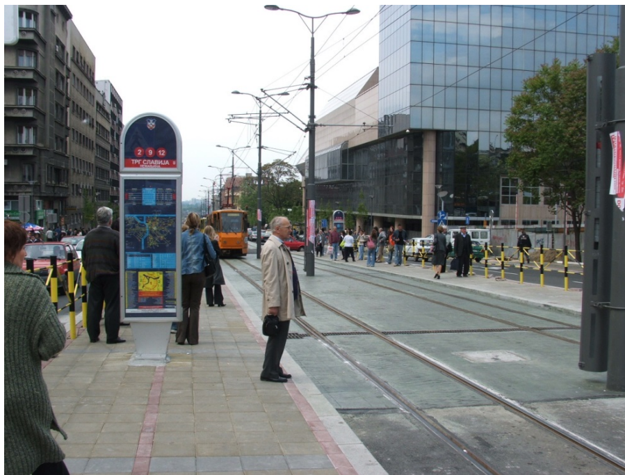
FIGURE 7 Modernization of tramway in Belgrade.
