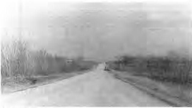
FIGURE 3 Type A aggregate-surfaced road (3).
