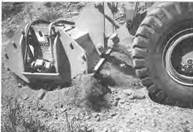
FIGURE 7 Roto Trimmer in operation; note small amount of dust and sidecast material.
