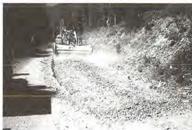
FIGURE 5 Roto Trimmer making first pass.
