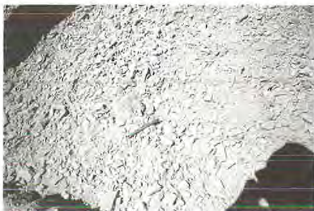
FIGURE 6 Typical road surfacing after being processed with Roto Trimmer.
