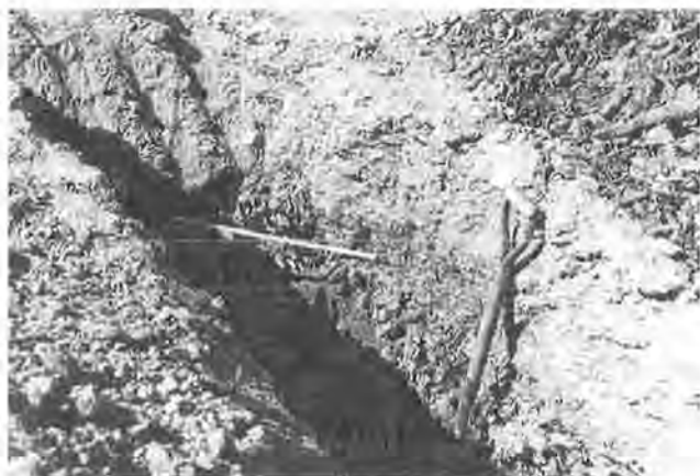
FIGURE 12 Base consisted of 20 to 22 in. of dirty gravel over \pm 8 in. of compacted tire chips; gravel was dry, whereas silty sand subgrade contained enough moisture to hold together when squeezed.
