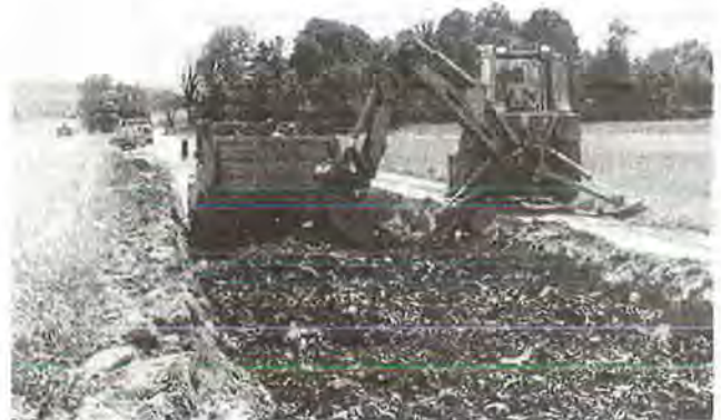
FIGURE 3 Leveling tire chips with backhoe.
