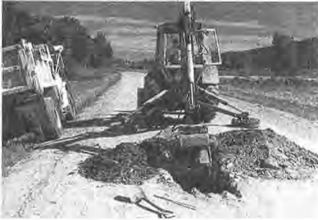
FIGURE 10 Excavating test pit in 1990 construction project.
