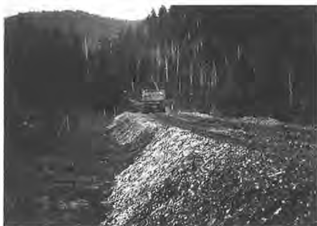
FIGURE 1 Unsurfaced woodwaste road.
