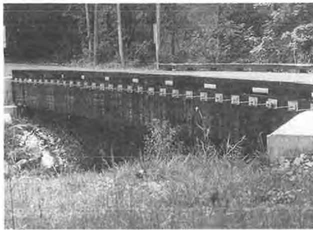
FIGURE 5 Camp Arrowhead bridge.
