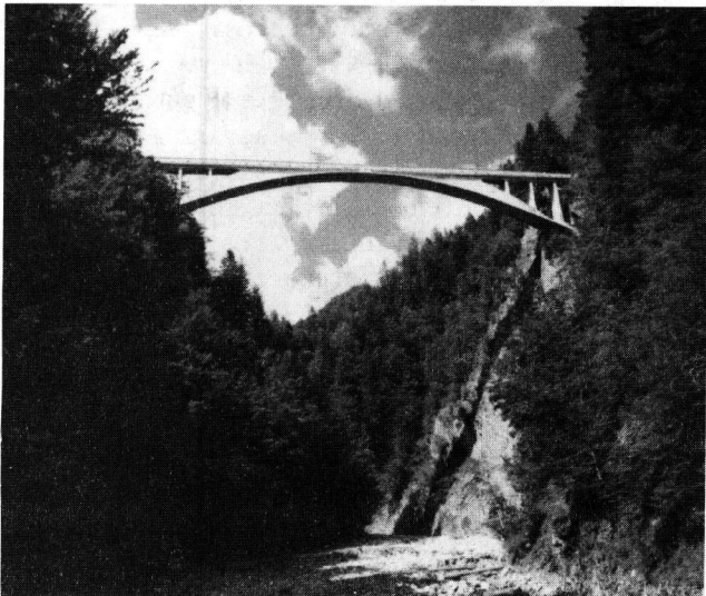
FIGURE 8 Salginatobel Bridge, Robert Maillart, Switzerland, 1930.
