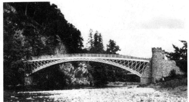
FIGURE 2 Craiglechie Bridge over Spey River, Thomas Telford, Elgin, Scotland, 1814.
