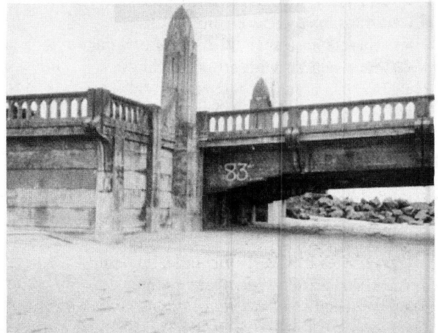
FIGURE 4 South abutment of first Alsea Bay Bridge showing concrete pylons.
