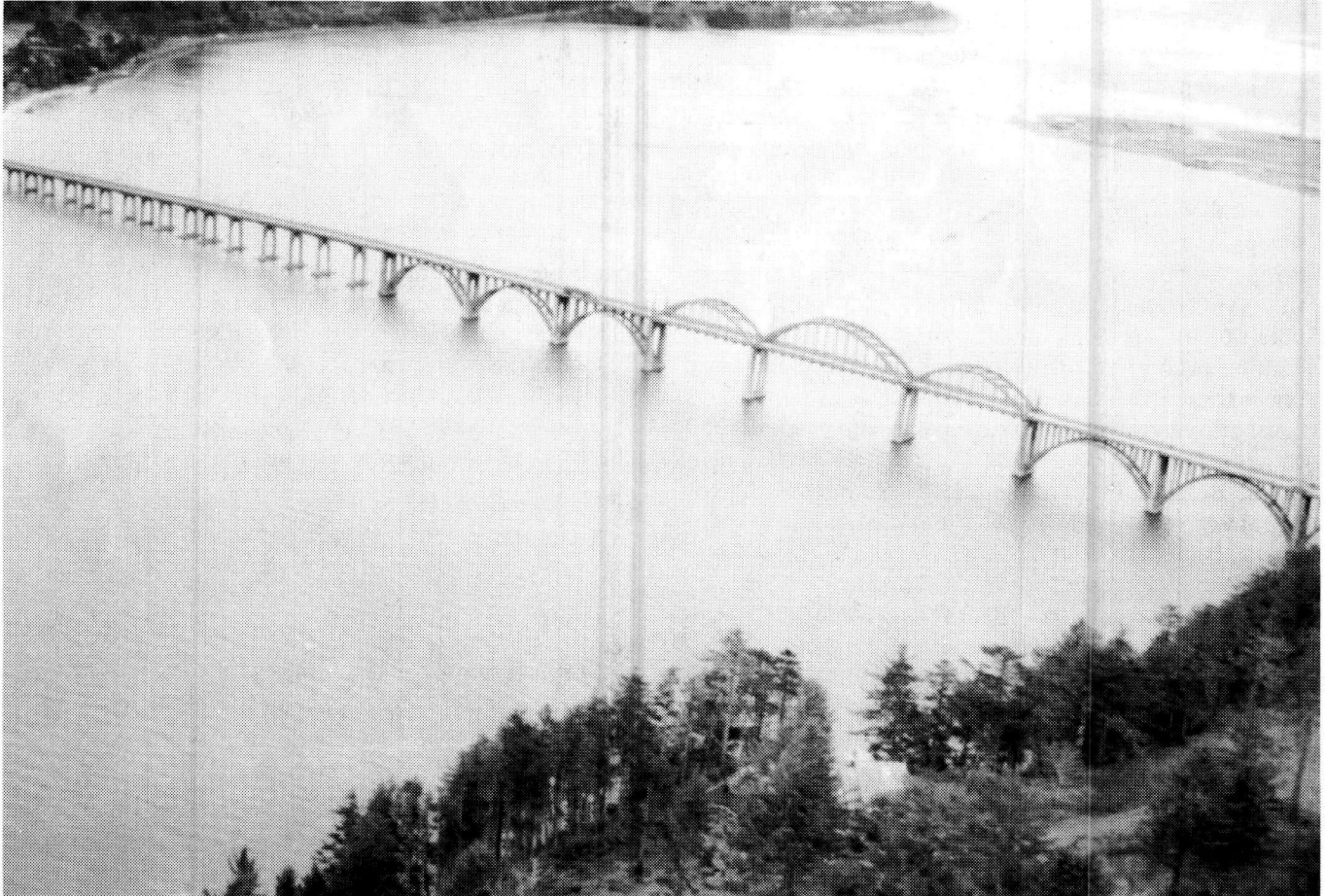
FIGURE 2 First Alsea Bay Bridge (looking southwest).
