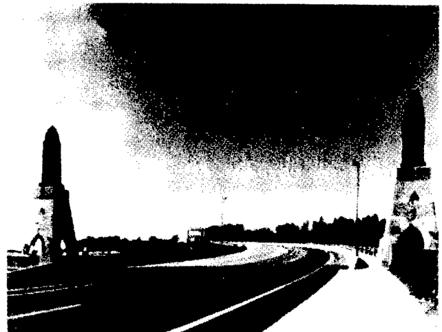
FIGURE 8 Bridgehead at south abutment.
