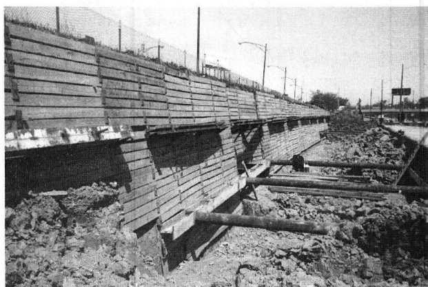
FIGURE 6 Soldier piles retained with soil anchors.
