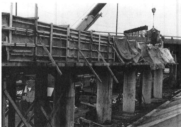
FIGURE 5 Job-built formwork.
