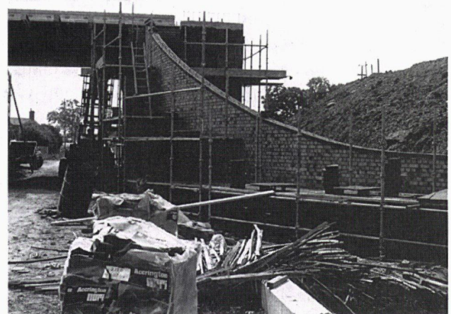
FIGURE 3 Foxcovert Road Bridge under construction.
