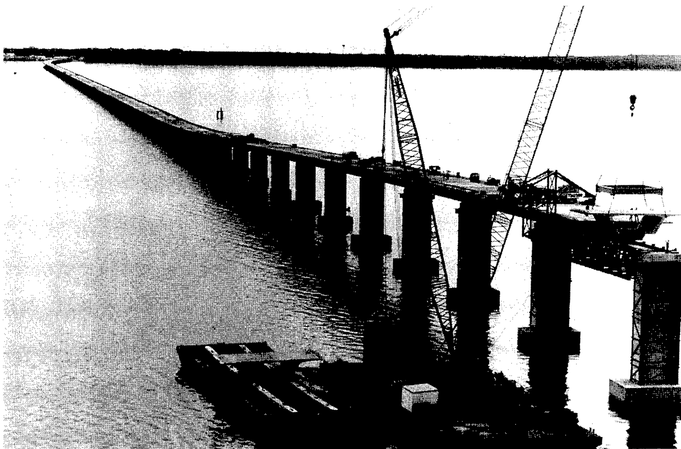
FIGURE 3 Typical 41.5-m (135-ft) spans were erected by span-by-span methods by using an assembly truss. The contractor was routinely able to erect four spans per week. During the week of September 20, 1992, the contractor was able to erect seven spans in 7 days [290 m (952 ft) of completed bridge in 1 week], a world record for span-by-span erection speed.
