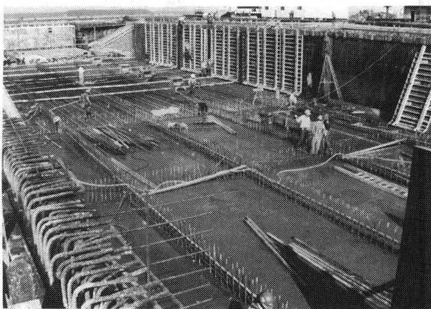
FIGURE 4 Completion of bottom slab and erection of wall forms.
