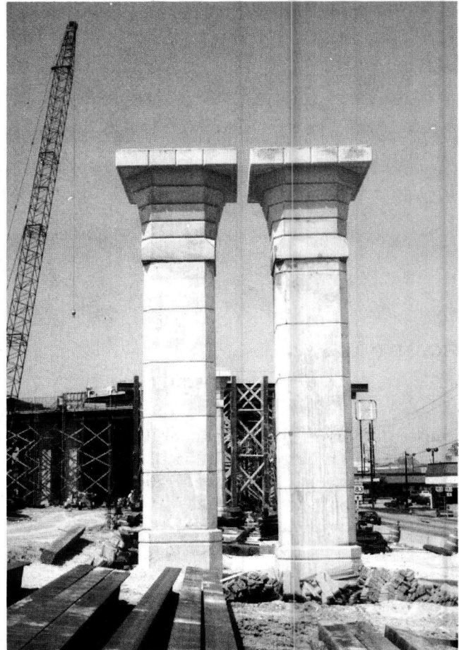
FIGURE 3 Small ramp piers in tandem to support flaring box girder.
