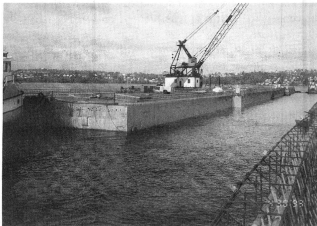
FIGURE 6 Pair of pontoons being maneuvered into position.
