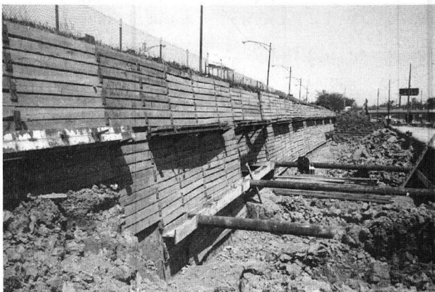
FIGURE 6 Soldier piles retained with soil anchors.
