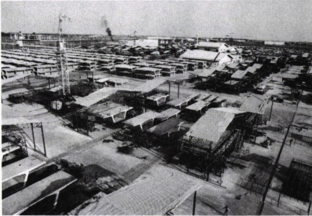
FIGURE 2 Aerial view of casting yard.
