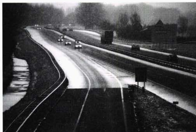
FIGURE 9 Evident difference in behavior of main road and shoulder (porous asphalt) and exit ramp (dense asphalt).
