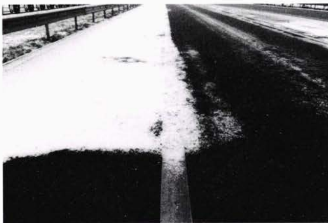
FIGURE 8 Hard shoulder of porous asphalt next to dense asphalt concrete road surface. Shoulder is fully covered with snow because without traffic action, salt remains in voids rather than transferring to surface.
