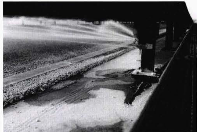
FIGURE 7 Sprinkler head spraying NaCl over bridge road surface.
