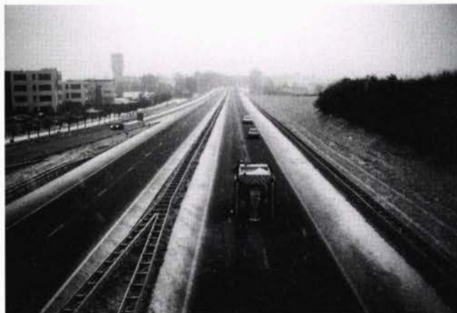
FIGURE 4 Prewetted salt is spread on surface before ice layer forms.
