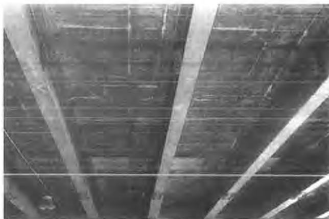
FIGURE 2 Underside of I-65 bridge.
