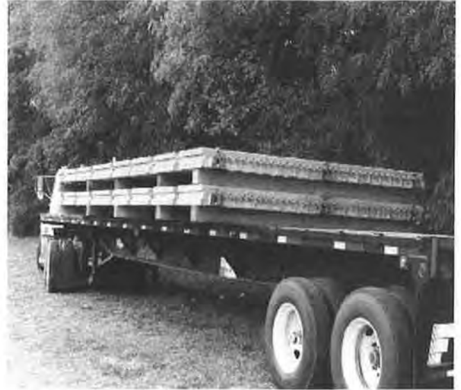
FIGURE 13 Exodermic panels in off-bridge staging area, Tappan Zee Bridge.
