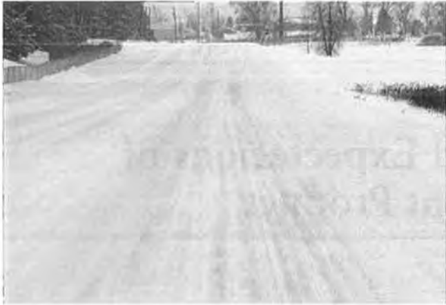
FIGURE 1 Snow-covered, compacted (worst).
