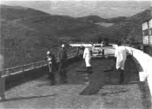
FIGURE 11 Applying deck primer—Caltrans's PPC overlay.
