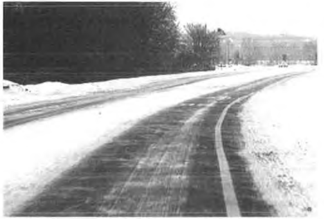
FIGURE 5 Two lanes plowed with centerline covered but edge lines showing.
