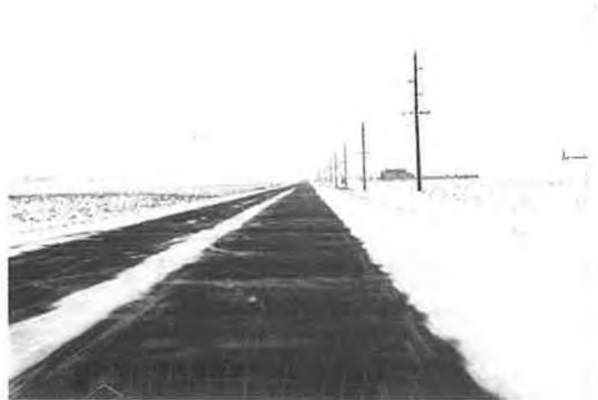
FIGURE 4 Two lanes plowed with centerline covered and no edge lines showing.
