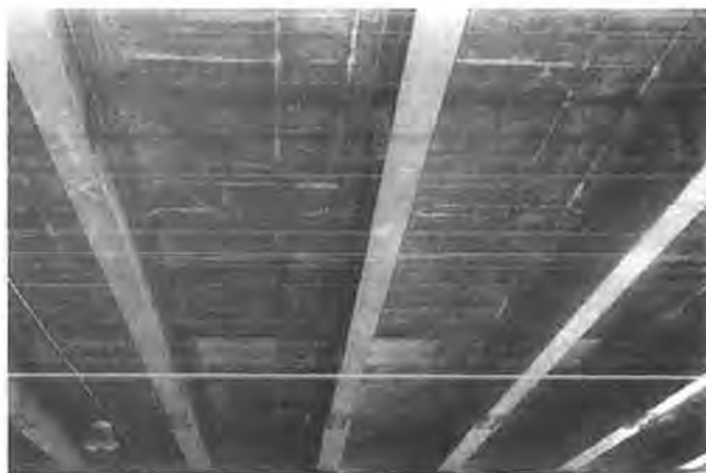
FIGURE 2 Underside of I-65 bridge.
