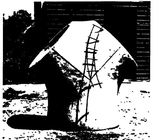
Figure 12. A single truss similar to those placed between circular wire-mesh cages in Pipe F.
