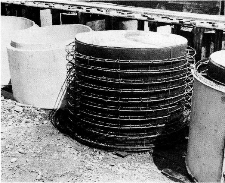
Figure 4. Reinforcing for Pipe B is shown in position.
