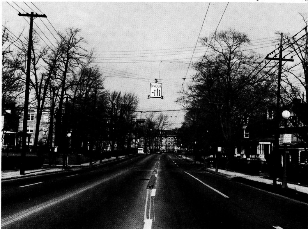
Figure 6. Reading and Gholson after improvements.
