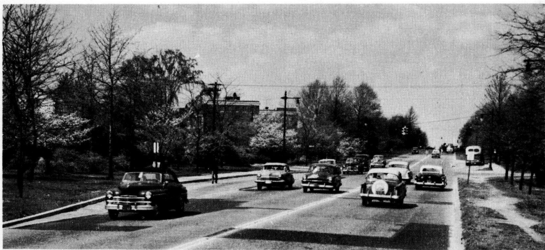
Figure 3. A level section of highway. The planting seen on the left insulates abutting properties from traffic noise. It serves the dual purpose of screening traffic from sight and sound. (Photo, courtesy of Bureau of Public Roads.)
