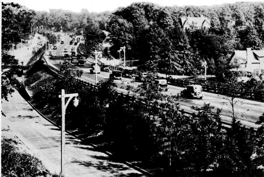
Figure 2. A raised section of highway. Abutting properties on the far side of the highway are well insulated from traffic noise by planting. (Photo, courtesy of Long Island State Park Commission.)
