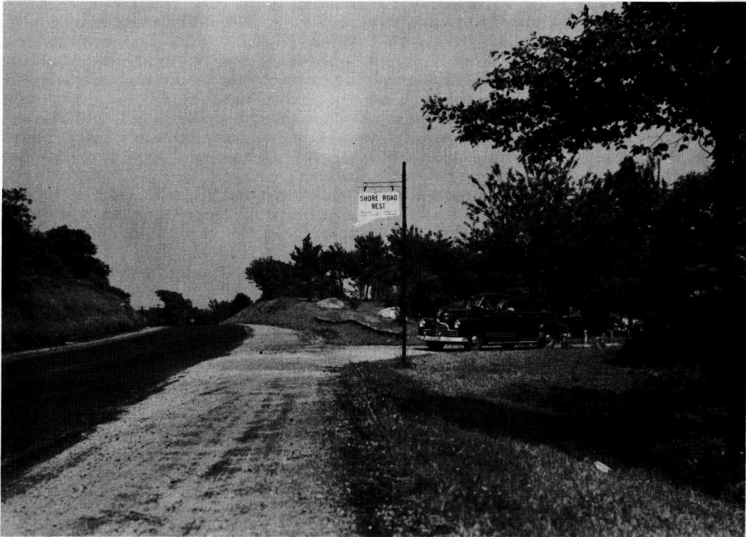
Figure 3. More parking turnouts and rest areas are needed along heavily traveled highways where motorists may relax, breathe fresh air, and ventilate their cars. Drivers welcome the chance to get away from traffic fumes and rest their eyes. This is an entrance to Shore Road Rest in Connecticut.
