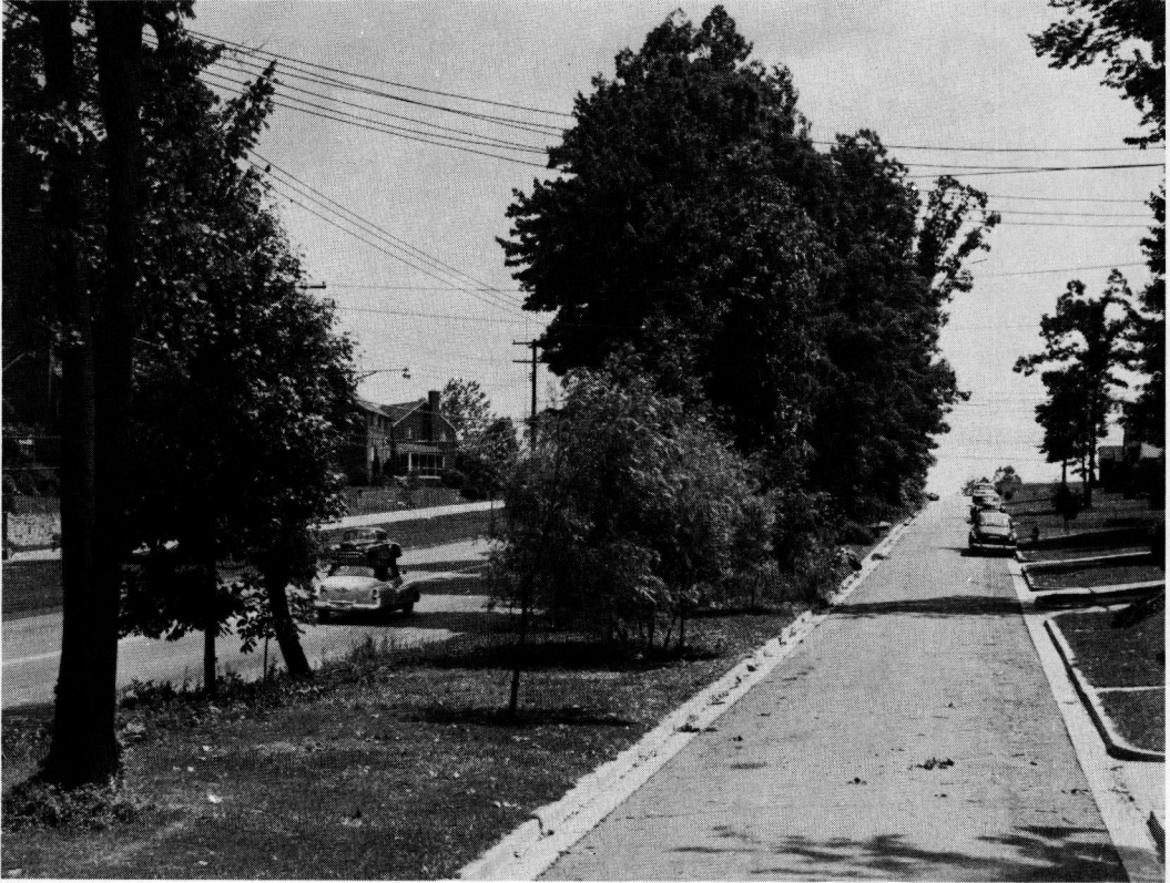
Figure 2. Frontage roads along this controlled-access highway increase the setback of buildings. Increased setback, together with a narrow buffer planting, reduces traffic annoyance to abutters.
