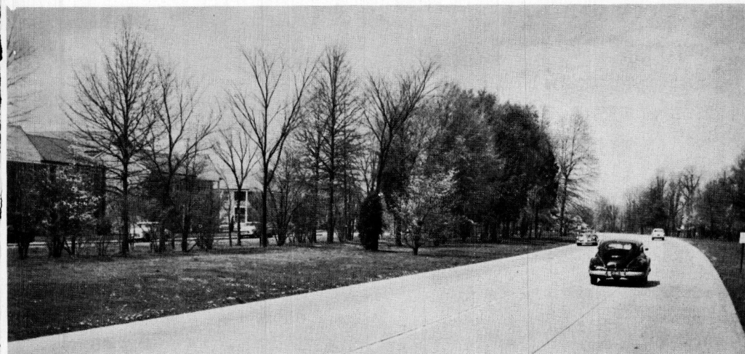
Figure 1. Planting of highway borders reduces annoyance of traffic to abutters. Liberal 75-ft. width between pavement and frontage road allows ample space for effective buffer planting.
