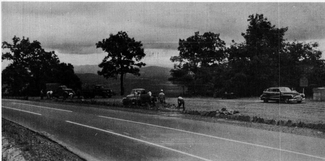
Figure 6. A parking turnout at a scenic overlook in historic Virginia. Note the separation of the parking area from the traveled way.
