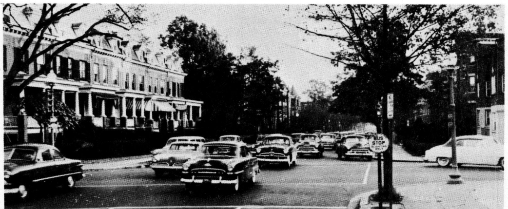
Figure 4. Looking south on Thirteenth Street during evening peak period - near Park Road with one-way traffic on Thirteenth Street.
