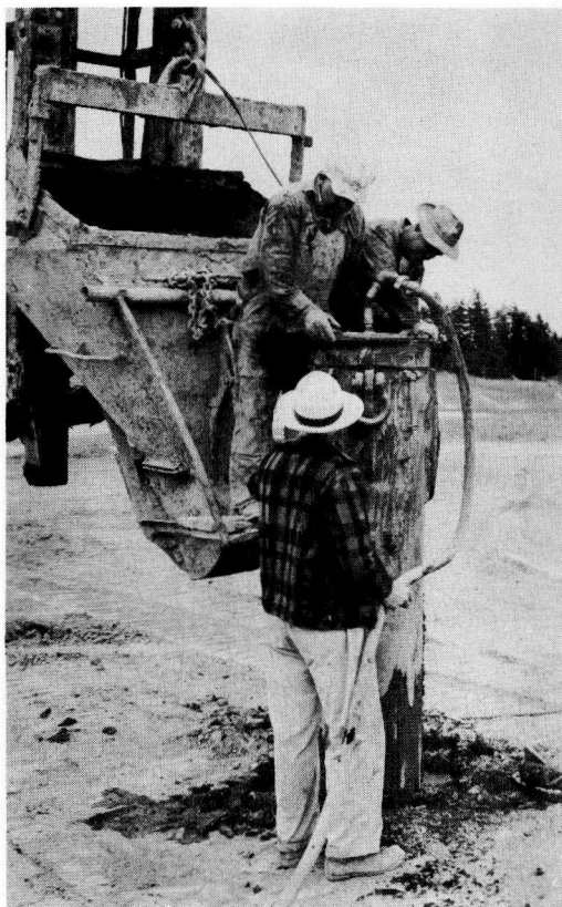
Figure 6. Clamping the air pressure cap on steel mandrel filled with \frac{1}{4} in. -0 drain material. Note the driving cap on the ground lower right.
