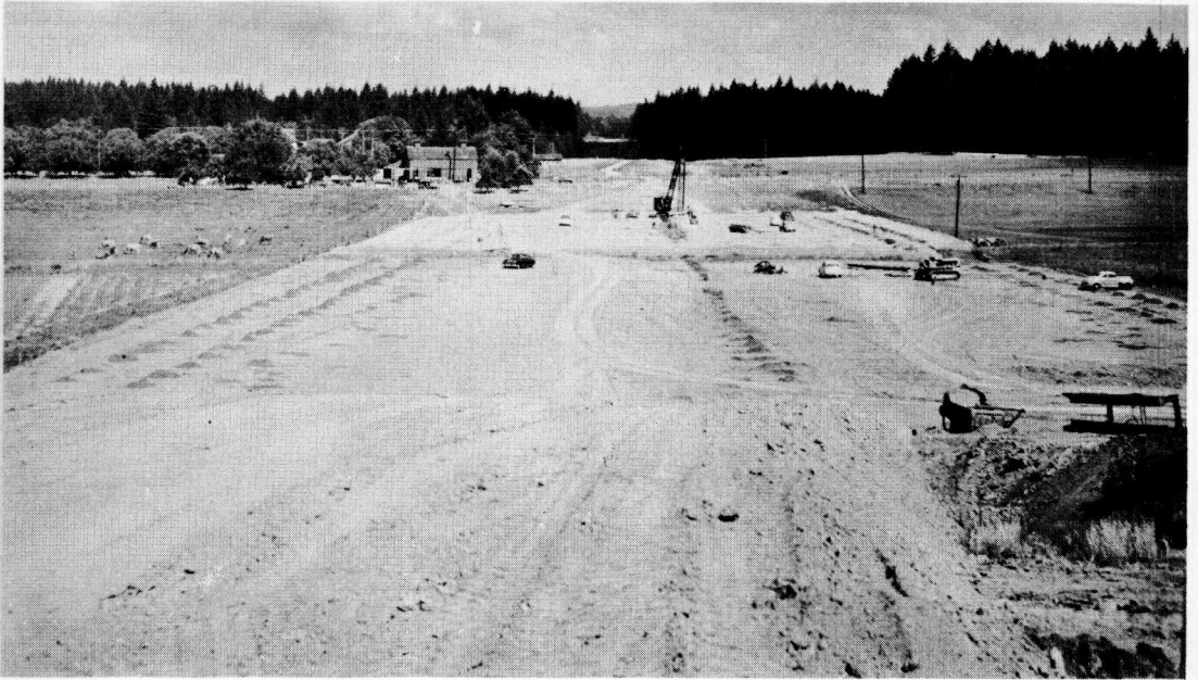
Figure 3. Working platform looking north, summer, 1952. Companion figure to Nos. 15 and 16. Pressure relief drain layout shown by excess \frac{1}{4} in. -0 drain material.
