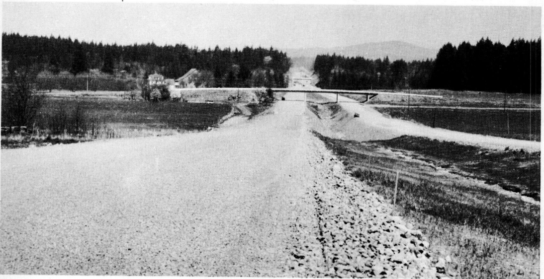
Figure 16. Looking north along west embankment just prior to placing asphaltic concrete paving. See Figures 3 and 15.
