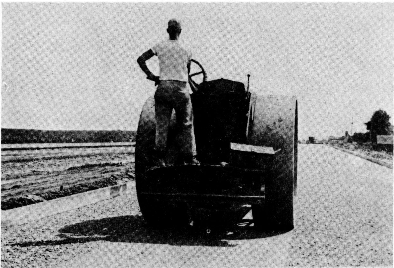
Figure 18. Texture of surface of open-graded stone subbase.
