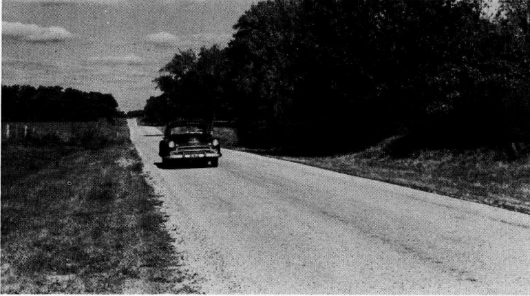
Figure 1. Soil-cement road after 18 years of service proves the dependability of the test procedures.
