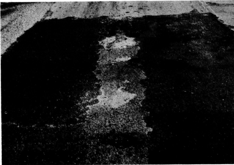
Figure 4. Condition of old pavement prior to resurfacing. View shows a pumping joint that has broken through an extensive bituminous patch.
