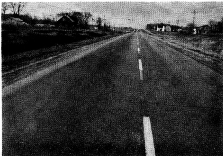
Figure 8. Typical condition of the resurfaced pavement December 1, 1954.
