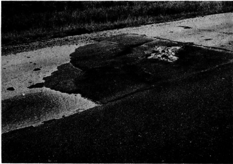
Figure 2. Condition of old pavement prior to resurfacing. Fore-ground example of extensive bituminous patching. Background example of numerous corner breaks.
