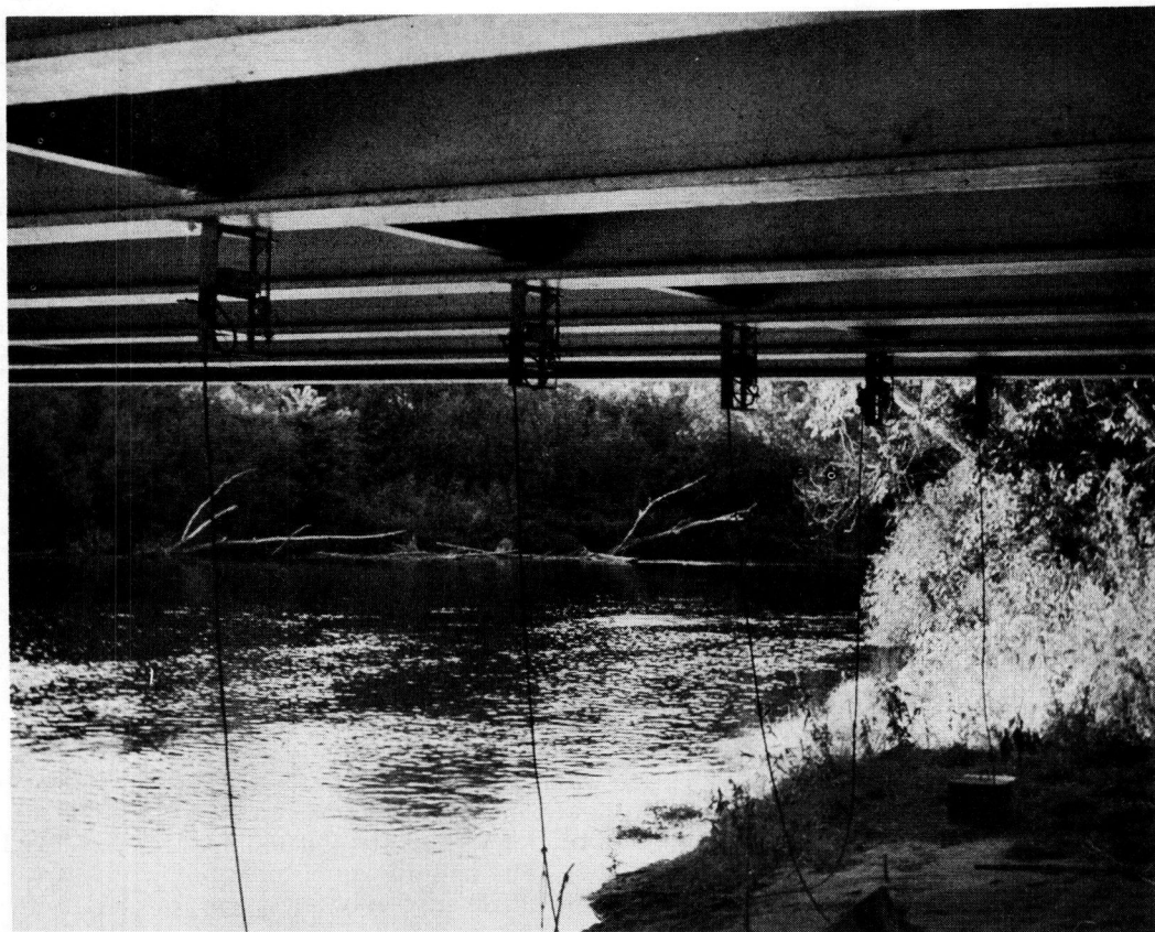
Figure 21. Deflectometer installation, Span 4.
