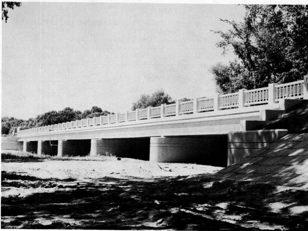
Figure 20. General view of Fennville Bridge.
