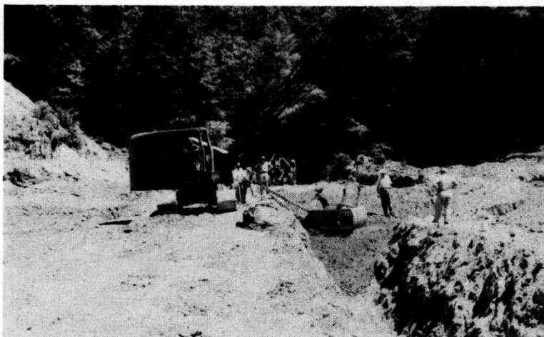
Figure 16. Refilling the imperfect ditch section with loose material. Facing north.
