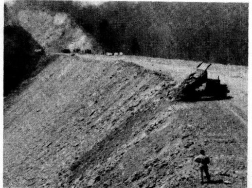
Figure 19. Final stages of end-dumped fill construction. Dressing of fill slopes. Facing west.
