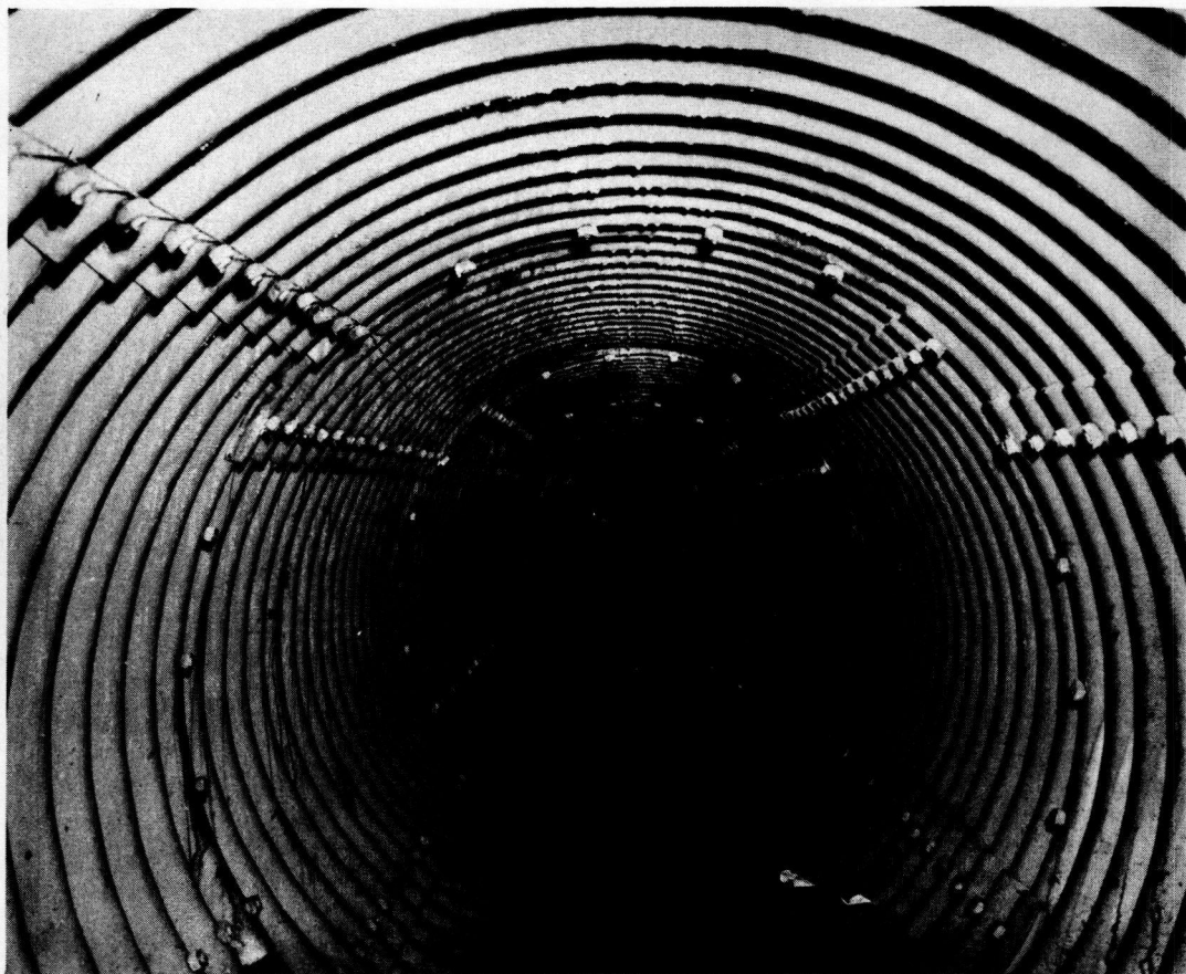
Figure 70. Pipe interior two years after installation.
