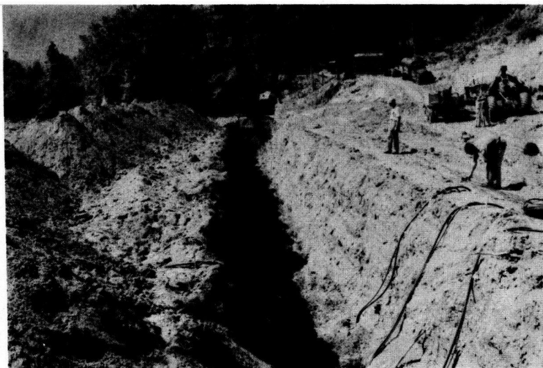
Figure 41. Installation of Ames settlement cells on the compacted fill mass adjacent to the top of the imperfect ditch.
