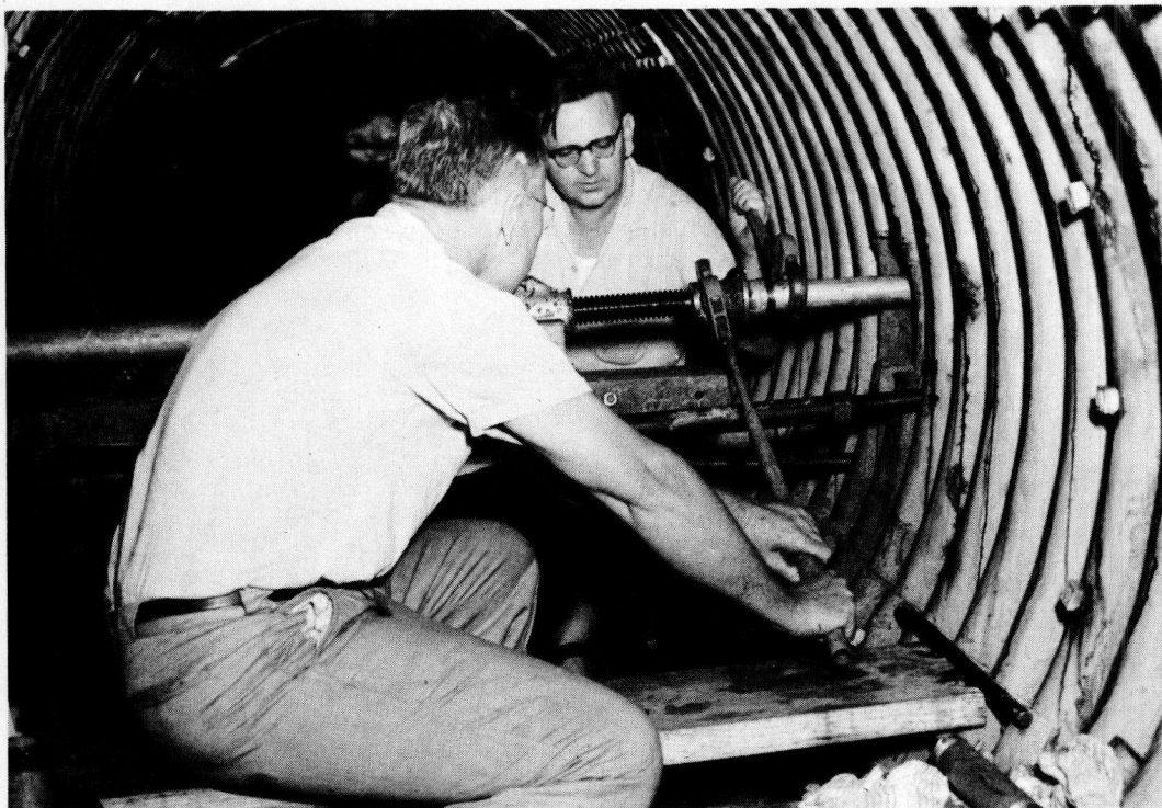
Figure 22. Forcing the sampling device into the side supporting material by means of a mechanical jack.
