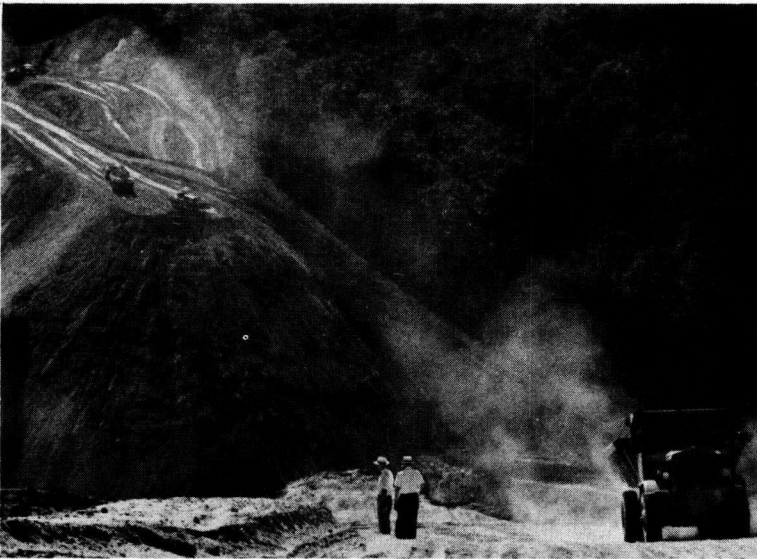
Figure 17. Construction of ramp by end-dumping from both eastern and western slopes. Facing west.
