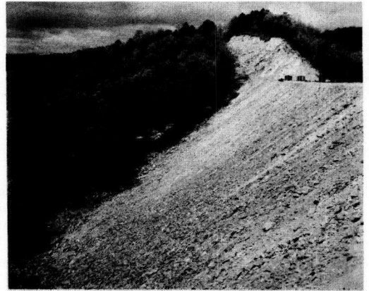
Figure 3. Completed fill covering culvert pipe used for experiment.
