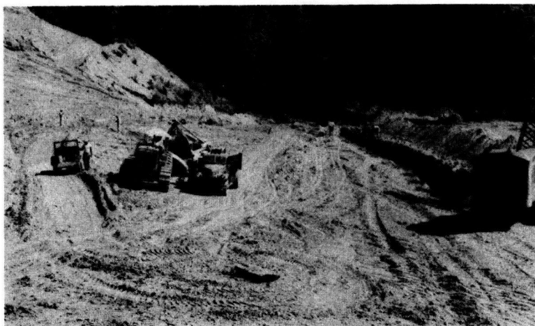
Figure 15. Cutting the imperfect ditch section on top of pipe. Facing north.
