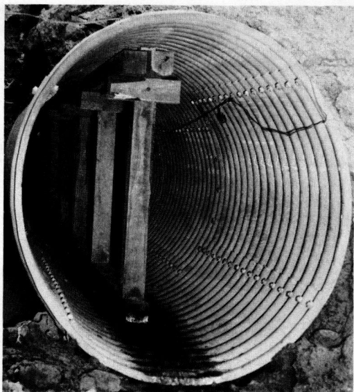
Figure 7. Pipe strutting. Electric line shown is for illuminating pipe interior.
