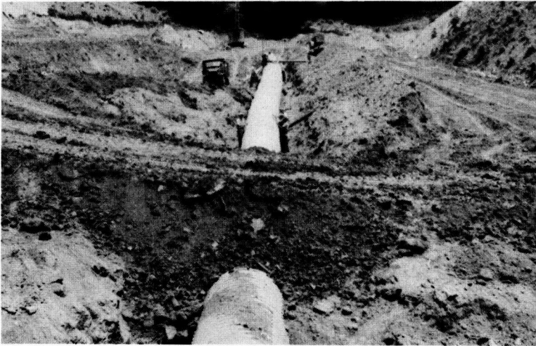
Figure 13. Removing slide material from immediate vicinity of culvert. Facing north.
