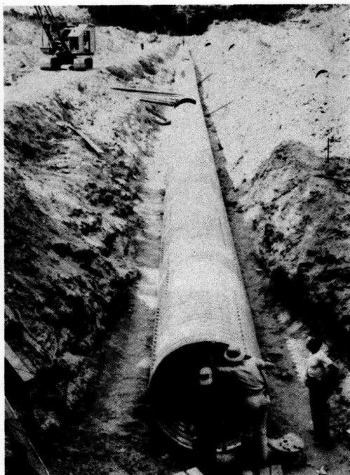
Figure 14. Culvert realignment after removal of slide material.
