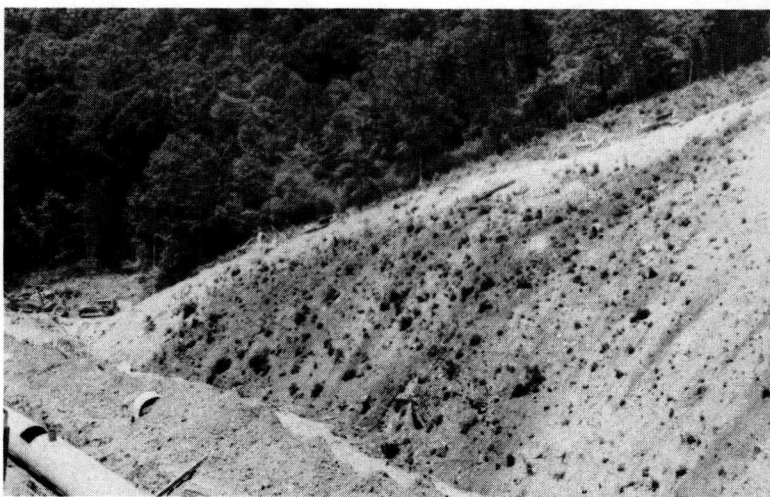
Figure 8. End-dumped material. Toe of western slope.
