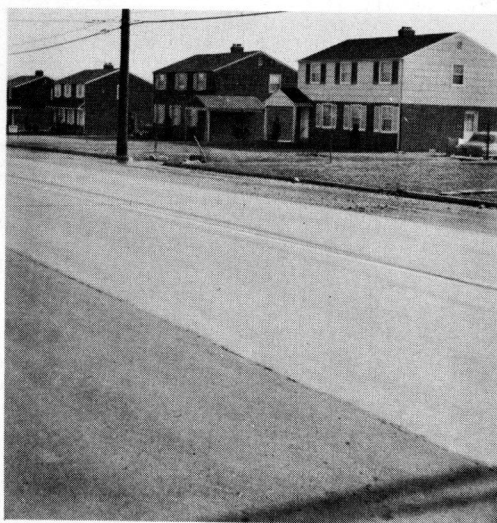
Figure 4. Route 422 shoulder - Lime-flyash-soil construction on shoulder opposite that given in Figure 3.
