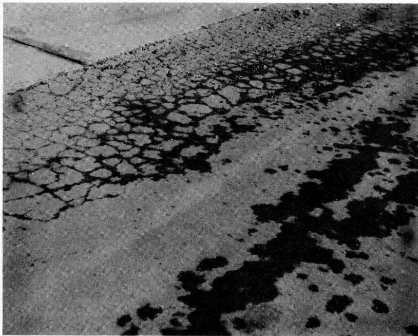
Figure 3. Route 422 shoulder - Break up of bituminous wearing course over stone base.
