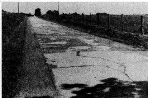
Figure 15 Albemarle County-Scottsville Area Poor performance of concrete pavement on soil derived from Triassic parent material.
