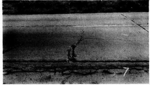
Figure 3. Random cracks.
