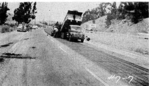
Figure 17. Paving over 3- by 8-inch mesh.
