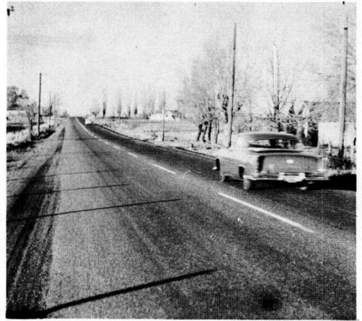
Figure 10. Resurfaced portland-cement concrete pavement with six inches of base added, in perfect condition seven years later.
