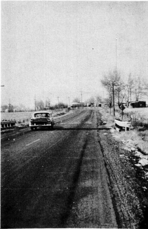
Figure 9. Traffic compaction of widened section, portland-cement concrete pavement, no base added over old pavement.
