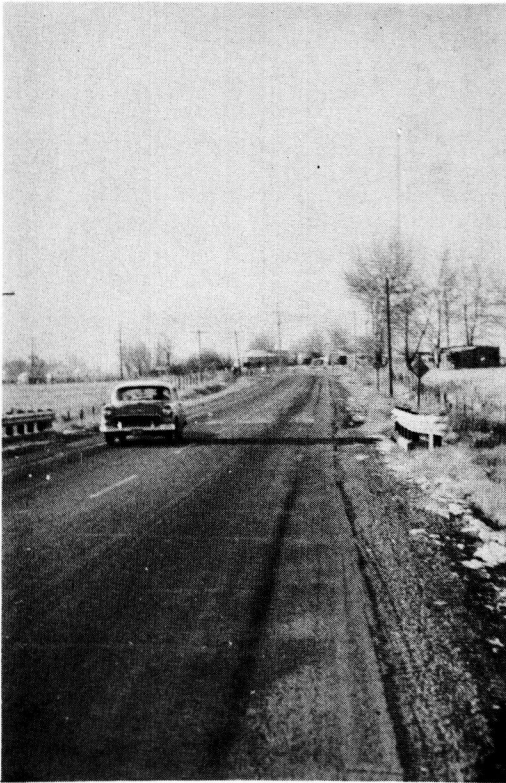
Figure 9. Traffic compaction of widened section, portland-cement concrete pavement, no base added over old pavement.
