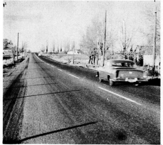
Figure 10. Resurfaced portland-cement concrete pavement with six inches of base added, in perfect condition seven years later.
