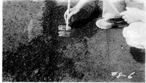
Figure 23. Position of fabric after completion of leveling course.
