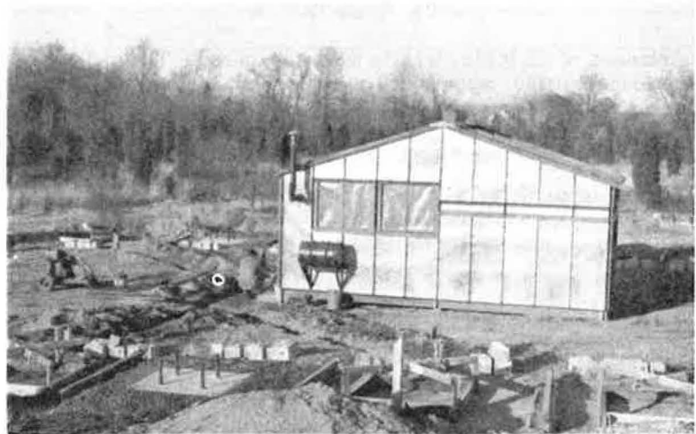
Figure 12. Preparation of soil installations. Wooden forms, completed slabs, installation of underground cables and the instrument building are shown.
