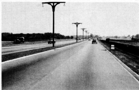
SITE NO. 12 — SOUTHERN STATE PARKWAY — 9 FT. WIDE GRASS MEDIAN WITH 3-INCH HIGH CURB.
