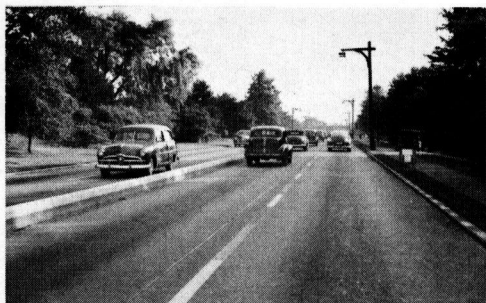
SITE NO.2 — SHORE PARKWAY — NARROW CONCRETE MEDIAN
