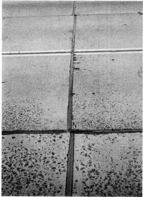
Figure 10. Sealed relief joint.
