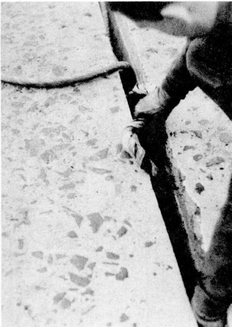
Figure 8. Paper rope being placed in relief joint.
