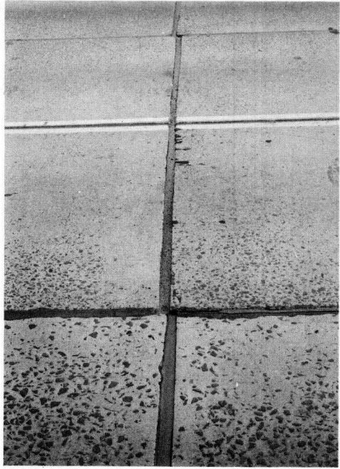
Figure 10. Sealed relief joint.
