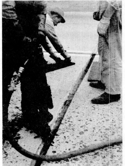
Figure 9. Special tamping device to level off joint filler.
