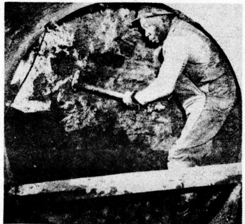
Figure 4. Excavation at Heading
